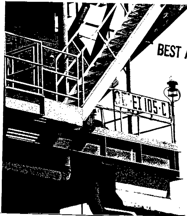
View of structure ID sign.
